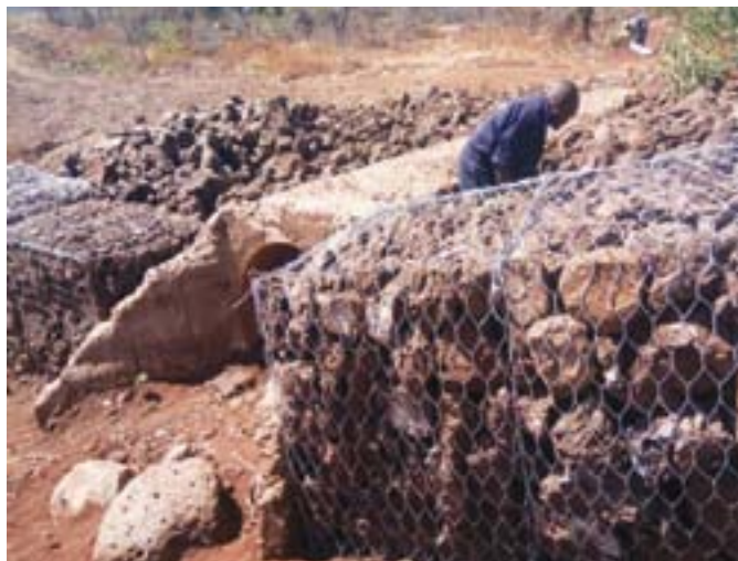
Kiirua Community Members participating in gabion construction at Kiirua valley in Meru County
