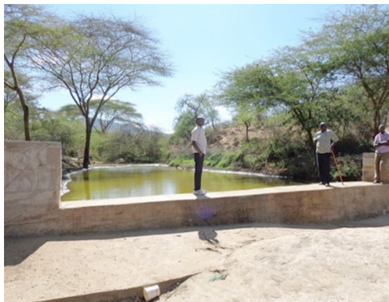
A completed sand dam holding water at Enkorika, Kajiado County
