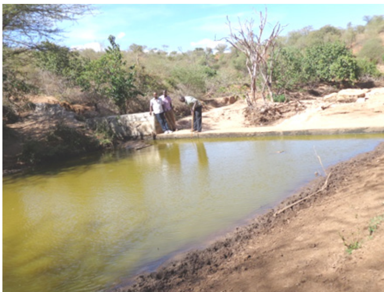
A completed sand dam holding water at Enkorika, Kajiado County
