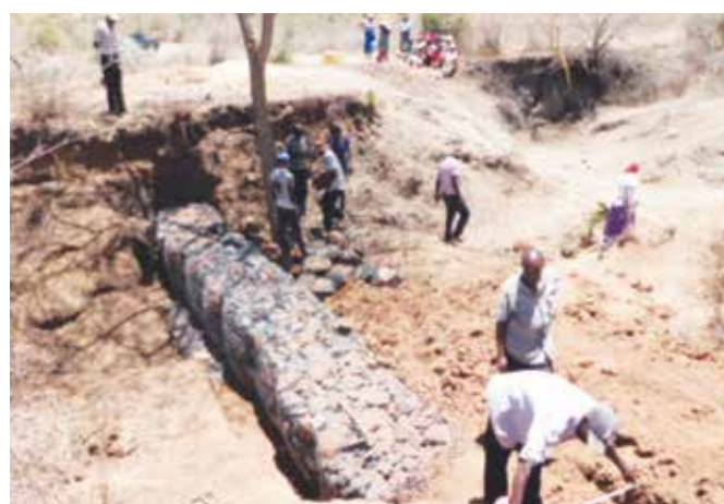
Construction work in progress
